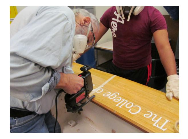
It took more than a little courage to cut through the beautiful Balsa Strip/Fiberglass Sandwich hull. It simply had to be shortened in order to accept the newly designed surface drive unit in production. The hull and drive unit combined would be just too long to fit into the Solar Splash rules.
