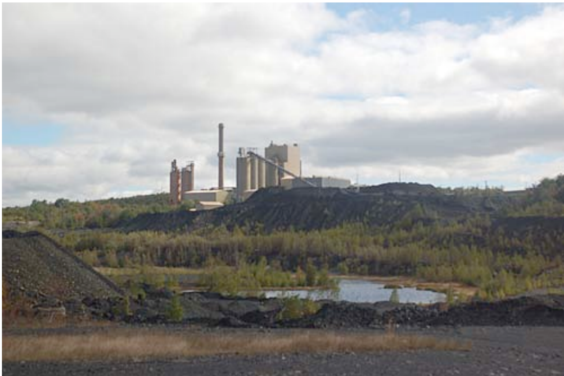
McAdoo Associates Superfund Site, Hometown, PA. Once owned by the Reading Anthracite Company and
