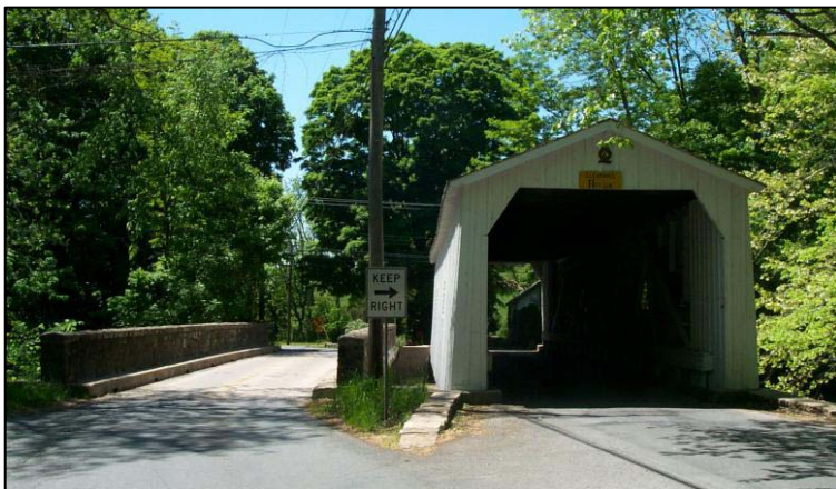
Green Sargeants Bridge, built in 1872. Located between Wickecheoke Creek between Sergeantsville and Rosemont From Hunterdon County Site
